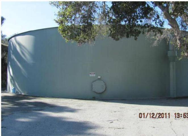
*Figure 2. The Ryan Ranch tank is a 500,000 gallon steel ground storage tank*
