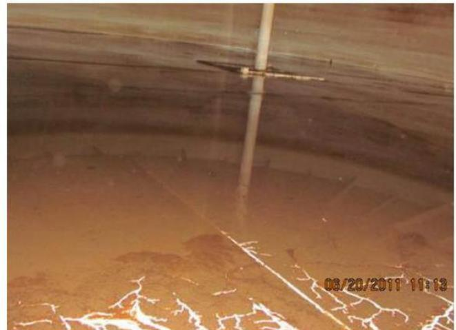
*Figure 3. Interior conditions of the Ryan Ranch tank prior to TRS.*
