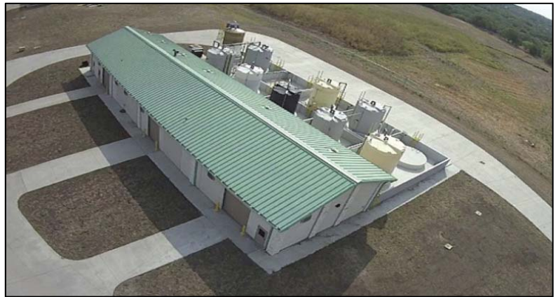
City of Midlothian Water Treatment Plant
