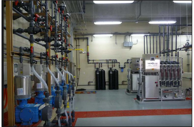
*Microclor® OSHG systems with Encore® metering pumps in foreground*
