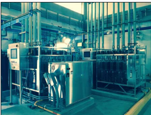
Three 1,500 PPD Microclor® OSHG skids
